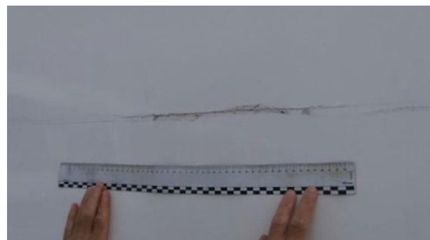
Side panels: Scratch with removal of material \geq 20\text{cm} within economic repair. Option to paint half panel
