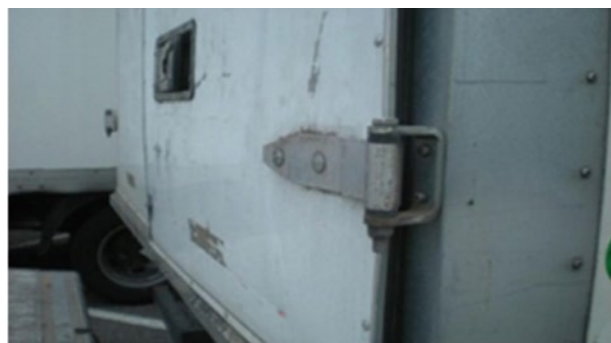
↻ Side and rear doors: Doors bent at fastening points for hinges, broken, perforated, or beyond economic repair
